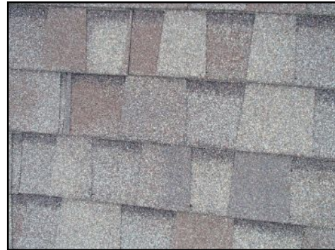
Shingles were in good condition
