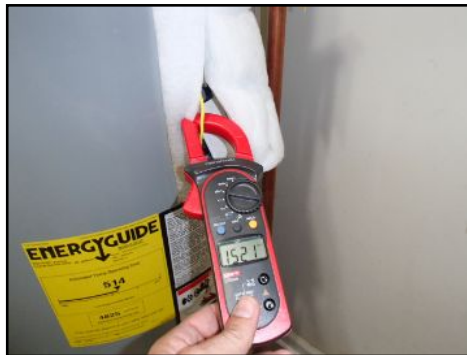
Upper element was operable
