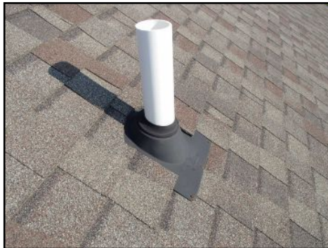
Plumbing boot was in good condition
